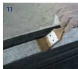
10 / 12 Illustrate the need to accurately cut the 450g/m² CSM strips 5mm narrower than the gap between the flange seal profiles. Wet out and laminate using 50mm brush and narrow roller.
