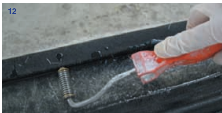
10 / 12 Illustrate the need to accurately cut the 450g/m² CSM strips 5mm narrower than the gap between the flange seal profiles. Wet out and laminate using 50mm brush and narrow roller.
