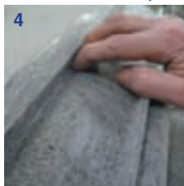
4 / 5. Butt joint the tissue, minimising the overlap and avoiding wrinkles.
