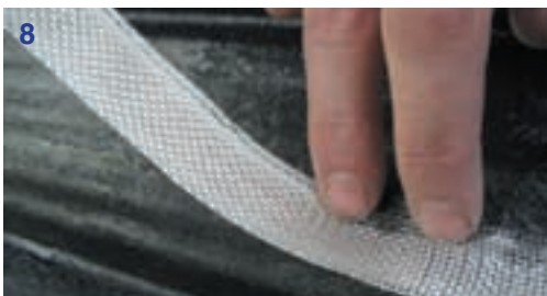
6 / 7 Use brush or roller to wet out and laminate tissue, using a minimum amount of resin. Do not use resin to flood the corners, instead gently work into the tissue. Do not over work the resin as this will lead to the splitting of the tissue layer.
