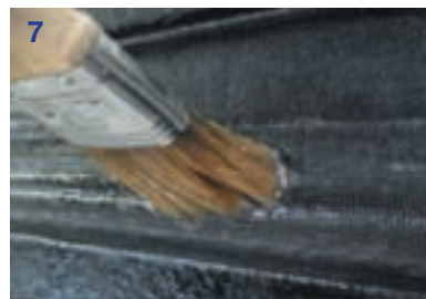
6 / 7 Use brush or roller to wet out and laminate tissue, using a minimum amount of resin. Do not use resin to flood the corners, instead gently work into the tissue. Do not over work the resin as this will lead to the splitting of the tissue layer.
