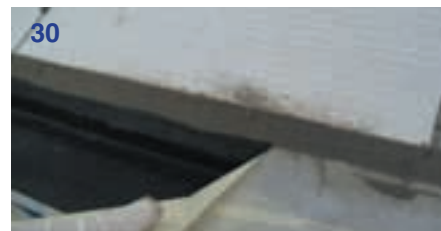
30 / 31 Remove the excess grout and neatly form a bevelled edge over the flow channel, and up to the masked edge. Remove the masking tape whilst the Fillite is still wet.
