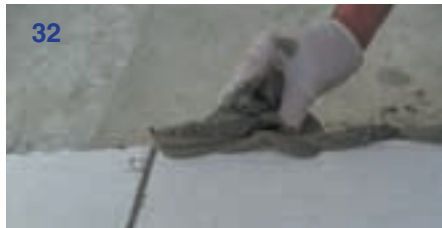
32 / 33 Complete the grout filling around the outer mould to form a neat edge as illustrated.
