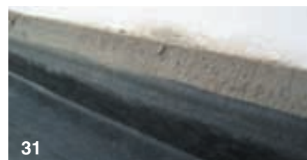
34 The Fillite now needs sanding to remove any high spots. Remove all dust.
