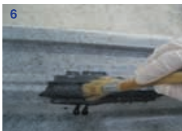
6 / 7 Use brush or roller to wet out and laminate tissue, using a minimum amount of resin. Do not use resin to flood the corners, instead gently work into the tissue. Do not over work the resin as this will lead to the splitting of the tissue layer.
