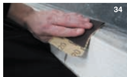
34 The Fillite now needs sanding to remove any high spots. Remove all dust.
