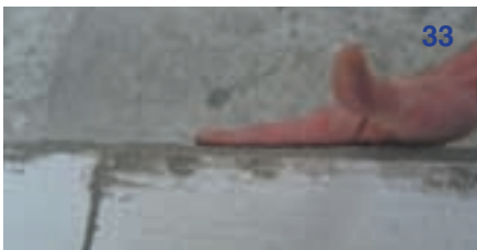
32 / 33 Complete the grout filling around the outer mould to form a neat edge as illustrated.
