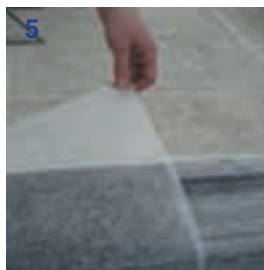
4 / 5. Butt joint the tissue, minimising the overlap and avoiding wrinkles.
